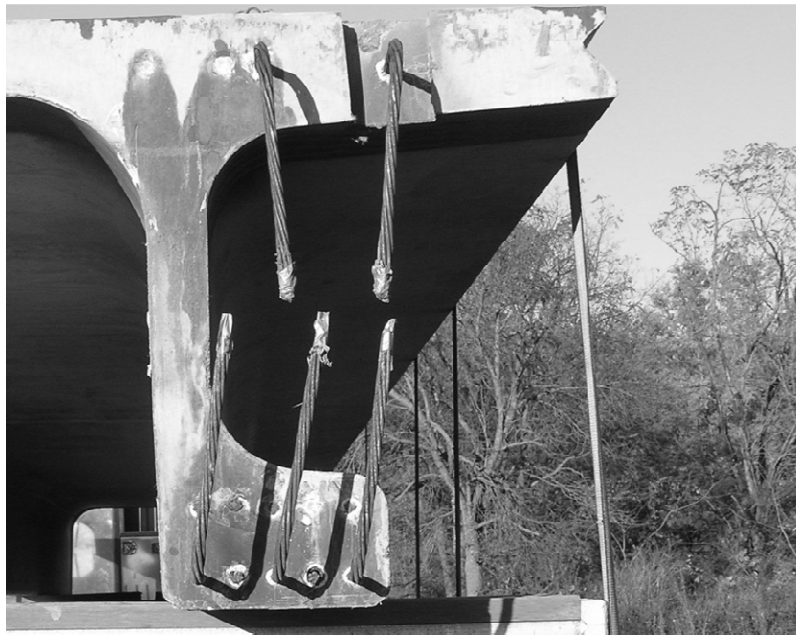
Figure 2.12-Pi-Girder Longitudinal Prestressing
