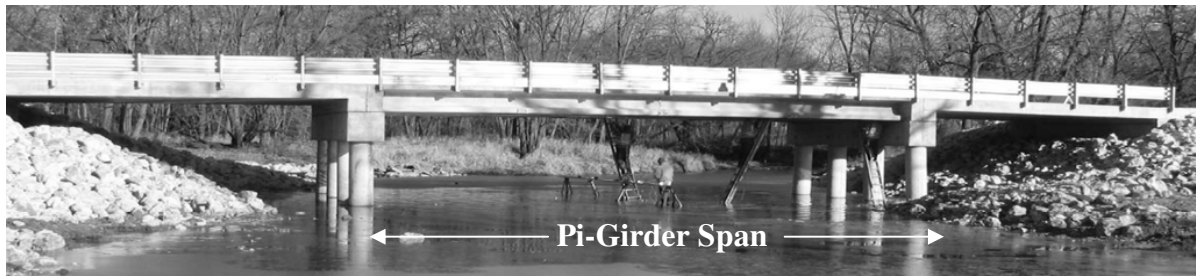
Figure 2.5-Elevation Photograph of Pi-Girder Bridge
